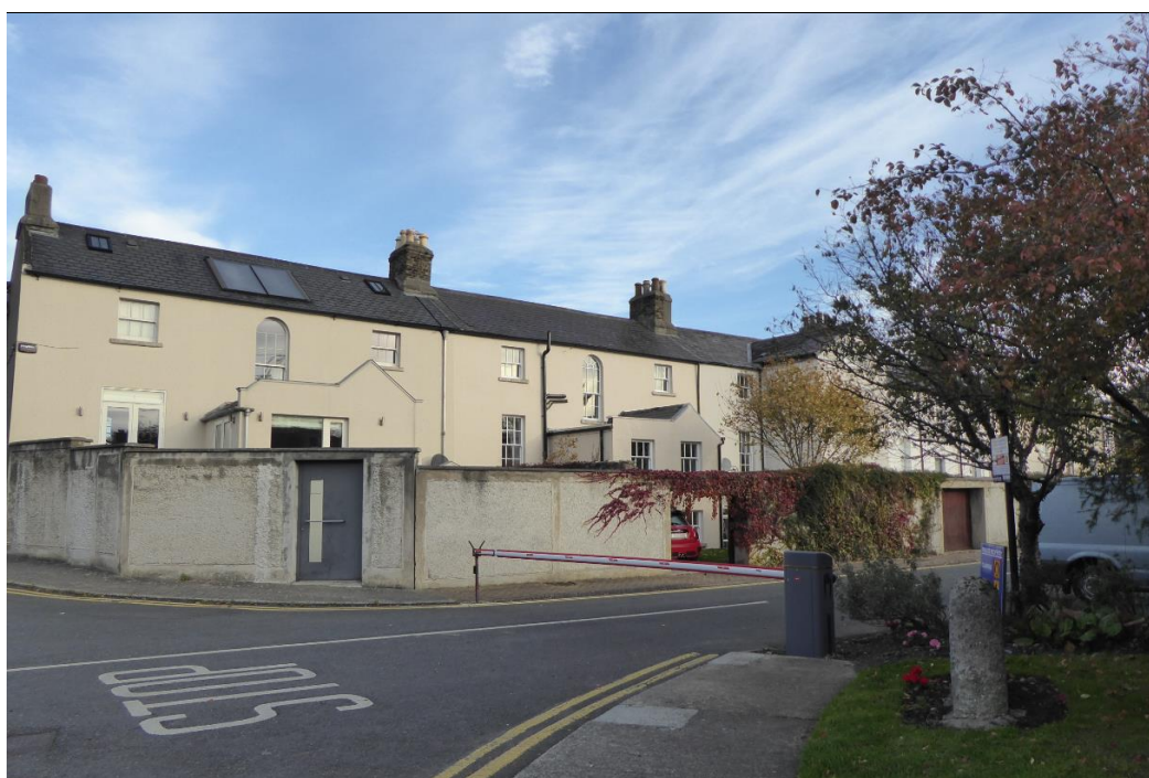
Plate 4.4 View of the rear of 8-16 Mt Merrion Avenue (even no's)
